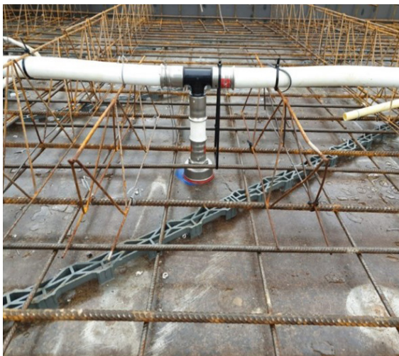
50P sprinkler holder glued to metal formwork
