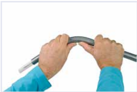
Bending with an external bending spring
