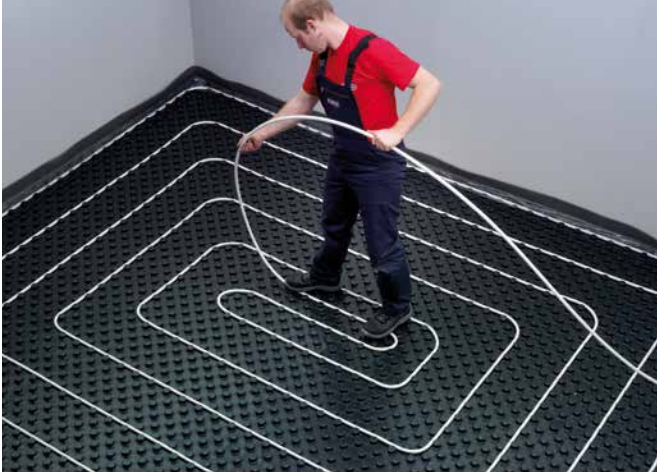
The pipe is laid in a spiral pattern .
