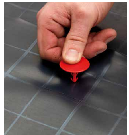
If desired, a sheeting tack can be used. This prevents the sheeting moving during the work.
